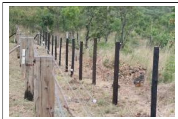
Fig. 6: The upgraded boma with the double electrified elephant proof perimeter fence
